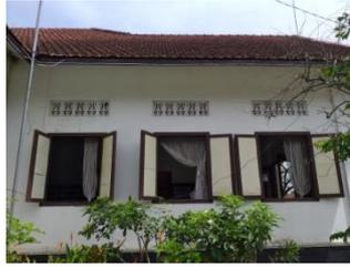
**Gambar 8. Sun Shading**
